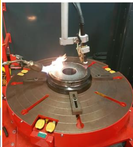
Pre-heating prior cladding
